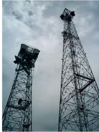
Figure 21: Steel tower structures requiring line-line intersections to compute center coordinates based on coordinates observed on each tower leg.
